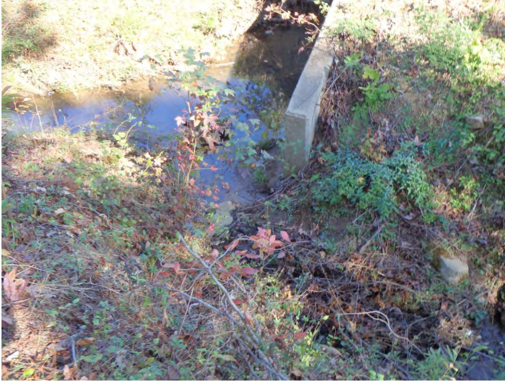
Photograph 15. Upstream view of S-5 at United States Highway (US) 41 crossing.
