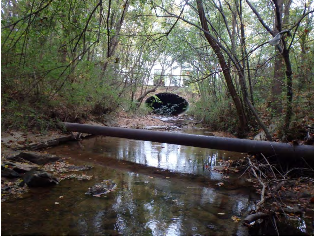
Photograph 29. Upstream view of S-14.
