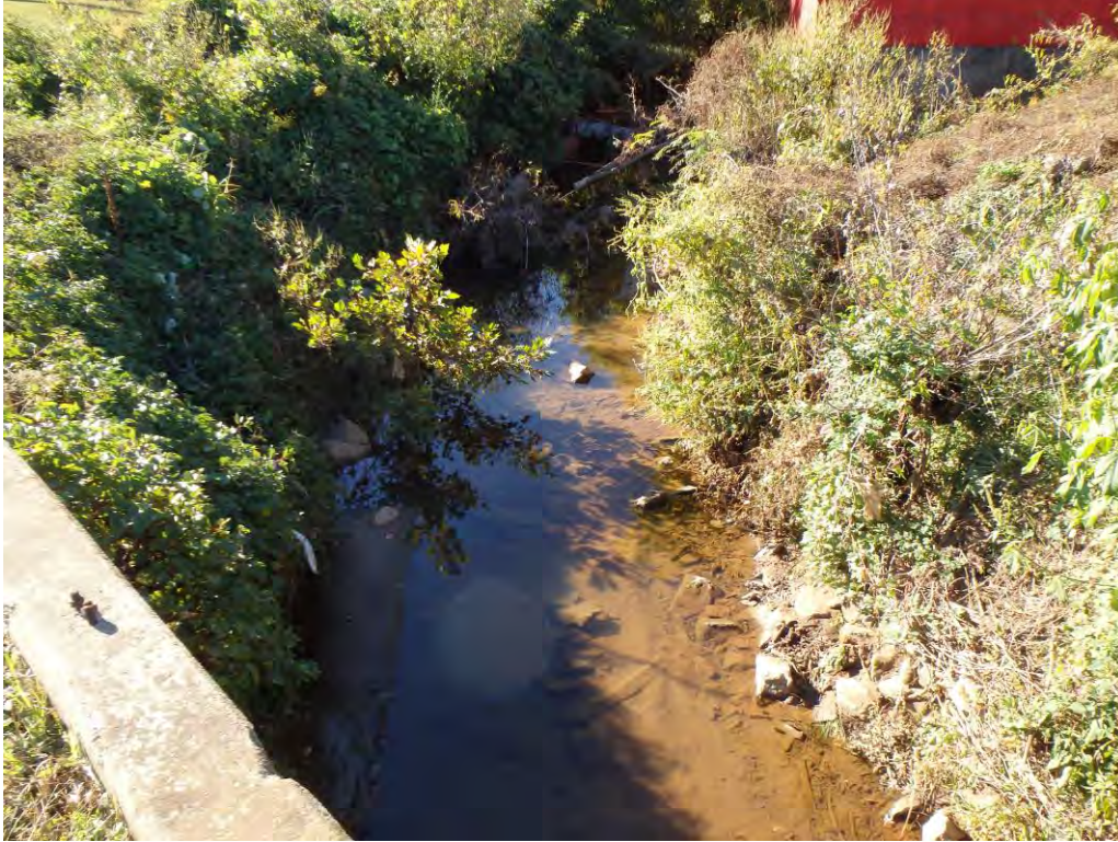
Photograph 21. Upstream view of S-9.
