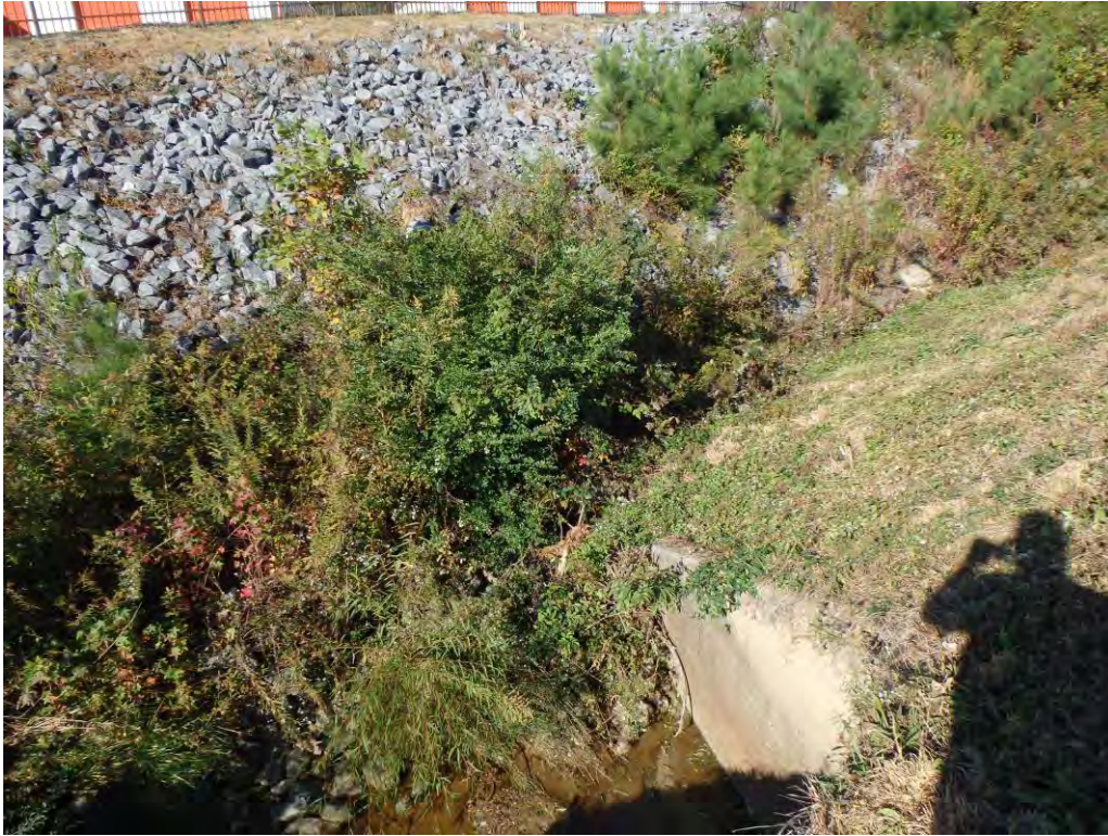
Photograph 23. Upstream view of S-10.
