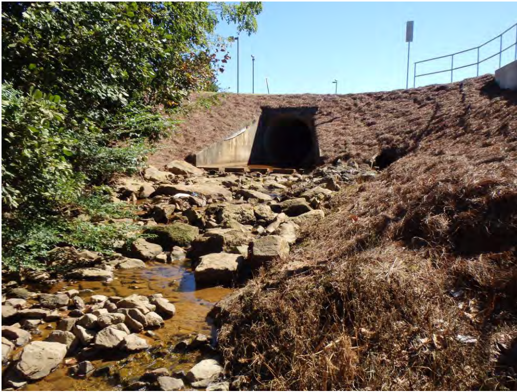
Photograph 7. Representative view of S-4 (Alt).
