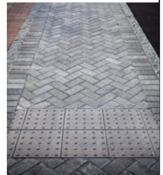
Crosswalk with Pavers
