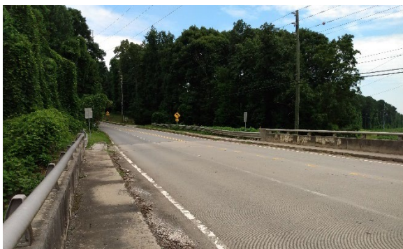
Sidewalks Along Hawkins Store Road Bridge
