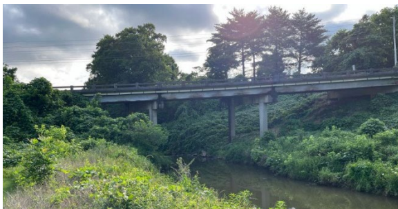
Bells Ferry Road Bridge Over Noonday Creek Programmed for Replacement
