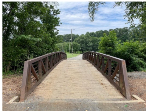
Existing Pedestrian Bridge Over Little Noonday Creek in Noonday Creek Park
