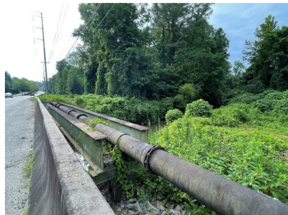
Water Line Crossing Noonday Creek South of New Chastain Road
