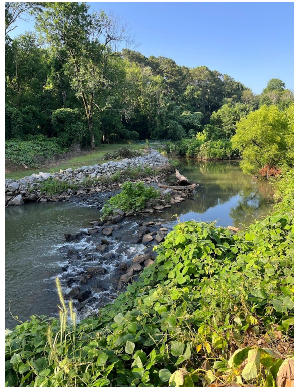
Noonday Creek As Shown From the Sewer Easement East of Bells Ferry Road
