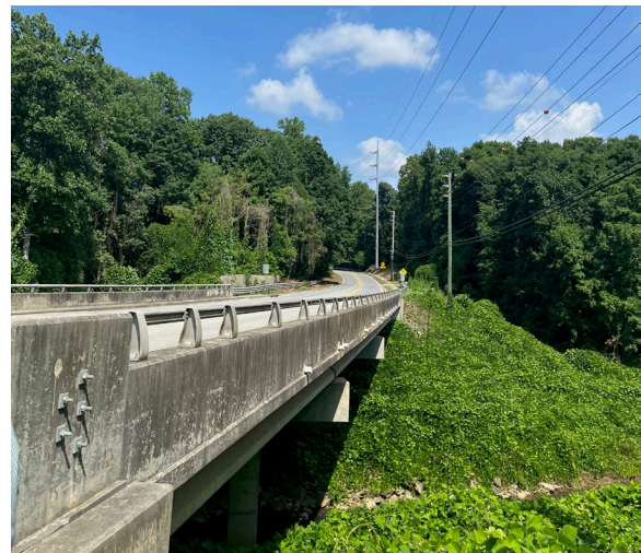
Blind Horizontal Curve Along Hawkins Store Road West of Noonday Creek
