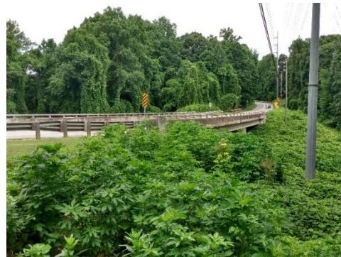
Bridge Over Noonday Creek, West Of The Noonday Creek Park Entrance
