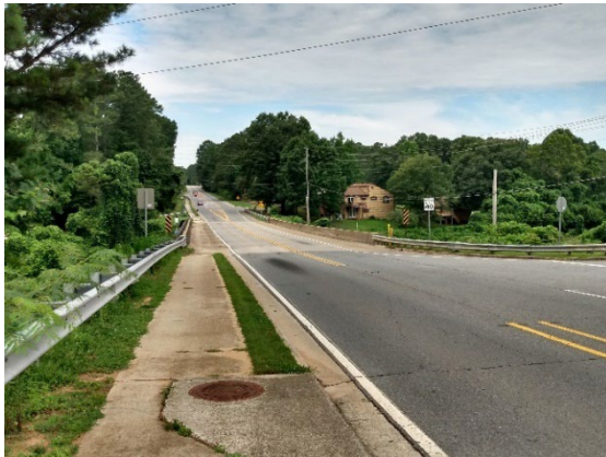
Shallowford Road Near Noonday Creek Includes Sidewalk on the South Side of the Roadway
