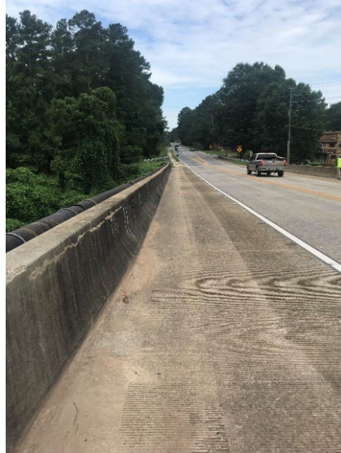
Bridge Contains Both Utilities and Wide Shoulders
