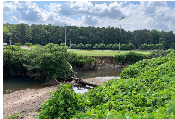
Bank Erosion Near Noonday Creek Park
