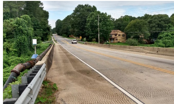
Looking West on Shallowford Road From Bridge Over Noonday Creek
