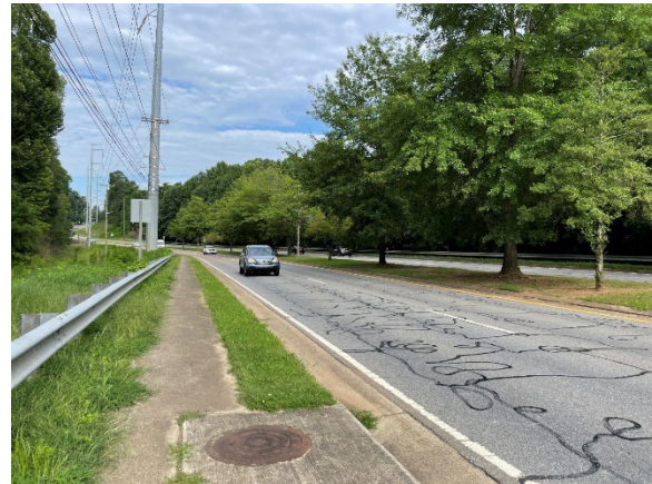
New Chastain Road West of Noonday Creek Trail
