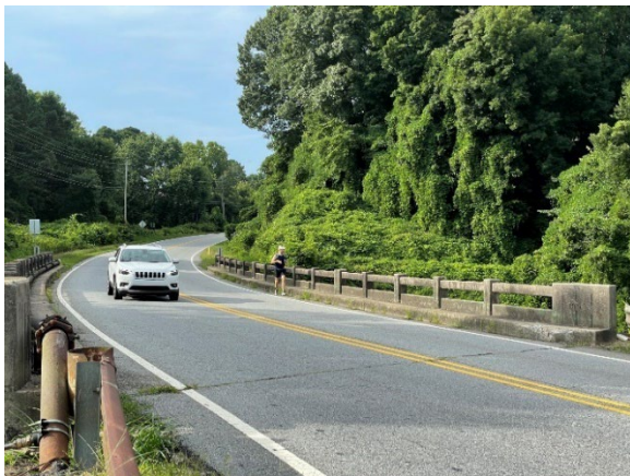
Pedestrian Jogging Along Bells Ferry Road on the Bridge Over Noonday Creek
