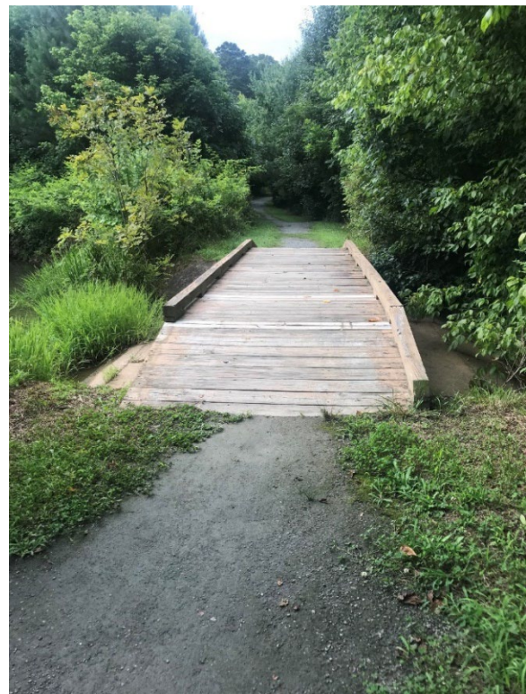
Boardwalk Within the Canterbury Greenspace
