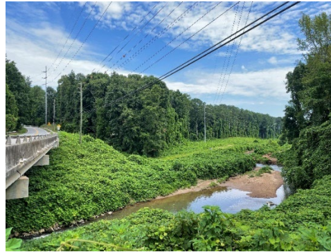
Overhead Utility Lines and Thick Vegetation North of Hawkins Store Road
