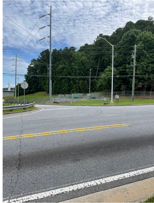
Entrance to Noonday Water Reclamation Facility Along Shallowford Road
