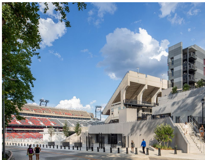
UGA Sanford Stadium Renovation Phase I | Athens
