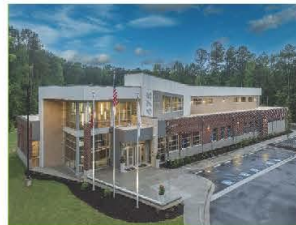
DISTRICT 4 RECREATION CENTER
